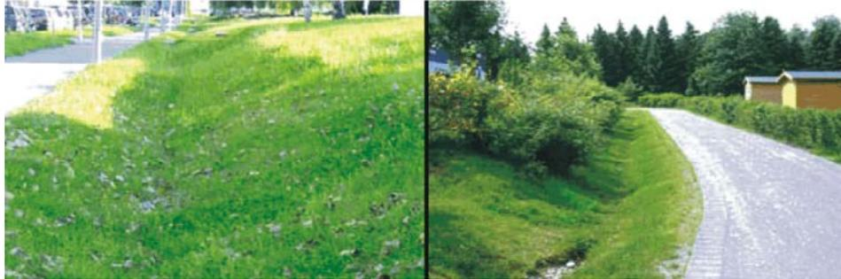
Fig. 3: Trench furrow infiltration in Germany [15]
